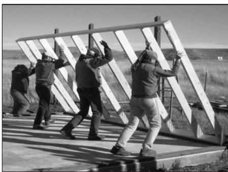
Raising the first wall of the storage shed
